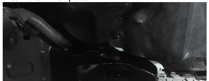
6: Finished weld, prep and paint surface while it's still warm.
